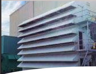
Intake & Filter Systems
